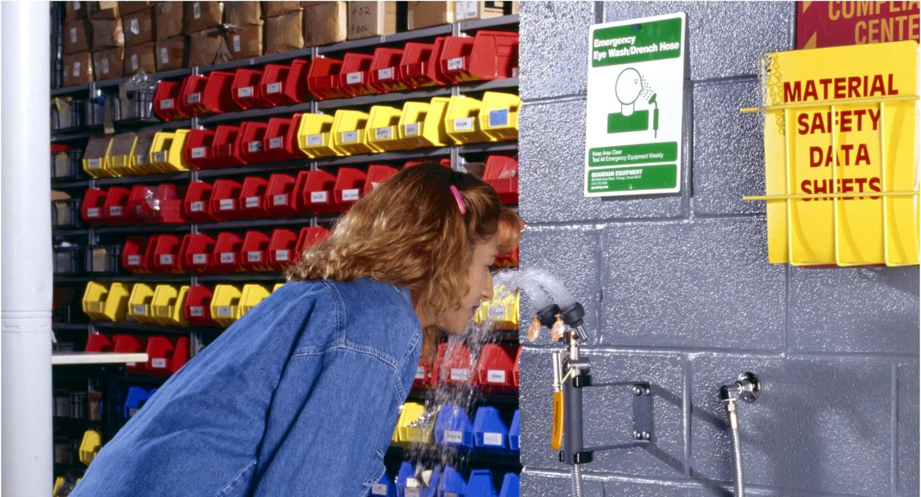
Standard emergency eye wash and shower equipment is constructed from a variety of materials, including stainless steel (shower pull rods and actuating arms), chrome plated brass (valves and eye wash components) and galvanized steel (pipe and fittings). In addition, standard units may include plastic components (shower heads, eye wash bowls, spray heads, etc.) that are molded from ABS, polypropylene and/or nylon.
