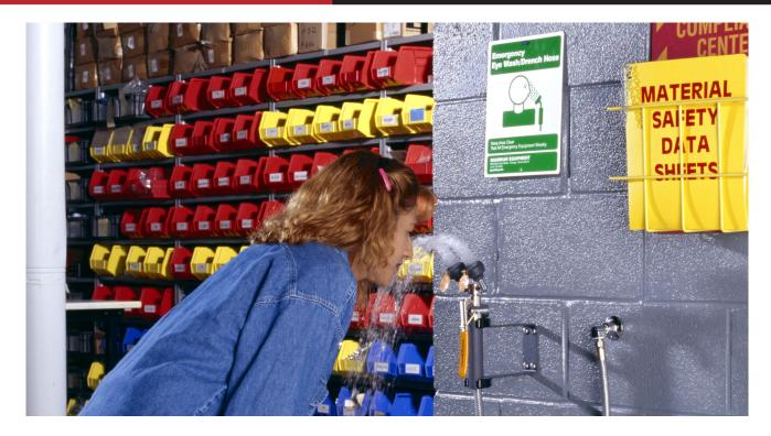
Standard emergency eye wash and shower equipment is constructed from a variety of materials, including stainless steel (shower pull rods and actuating arms), chrome plated brass (valves and eye wash components) and galvanized steel (pipe and fittings). In addition, standard units may include plastic components (shower heads, eye wash bowls, spray heads, etc.) that are molded from ABS, polypropylene and/or nylon.
